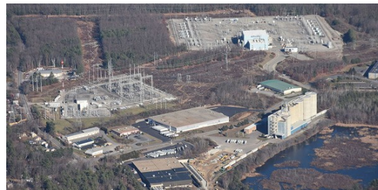
Substation in Ayer, Mass.
